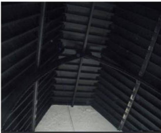
Figure 1 – inside view of existing roof
