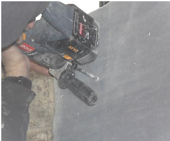
Drilling Spaceloft® - 40mm layer
